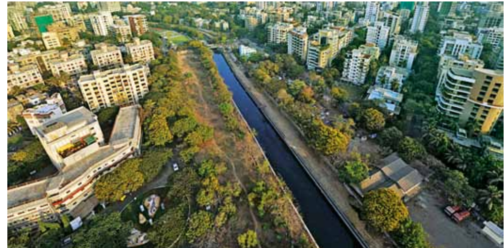
Top: Irla nullah overview in Juhu. Middle: Neglected and abused Condition before. Below: Visualisation post implementation of the project
